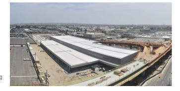
facility officially topped off in concrete in July as the last of 233,000 cubic yards of concrete were poured since breaking around in October 2019. The Intermodal Transportation
